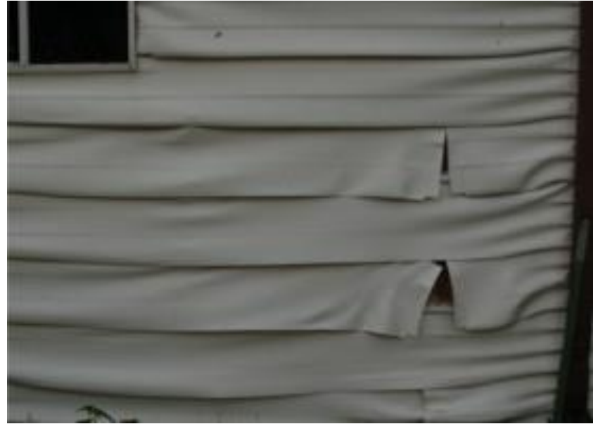
Cracked Siding
