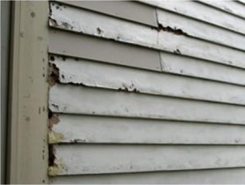
Rotting Siding
